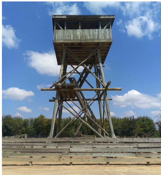
Figure 10: A fire tower built of wood materials
